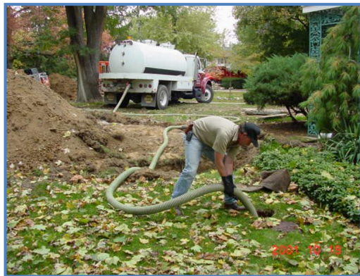
Septic System Pump-out
