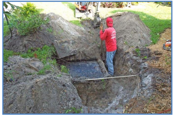
Septic System Repair
